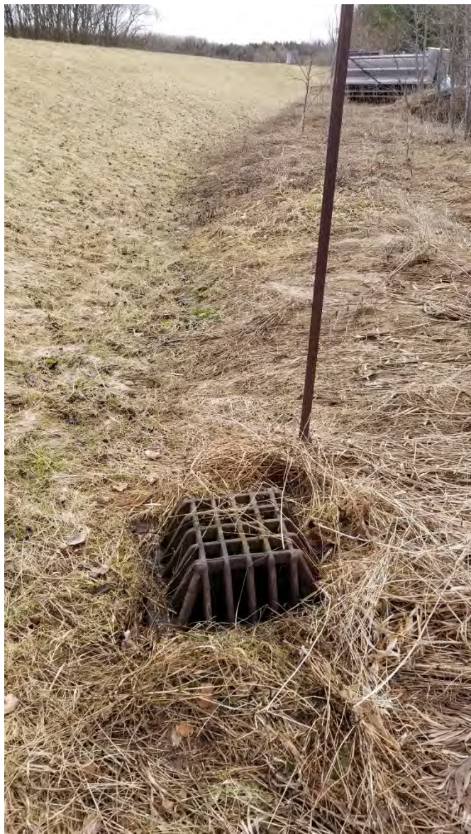
Land side of Dyke, Bird cage inlet from toe drainage
