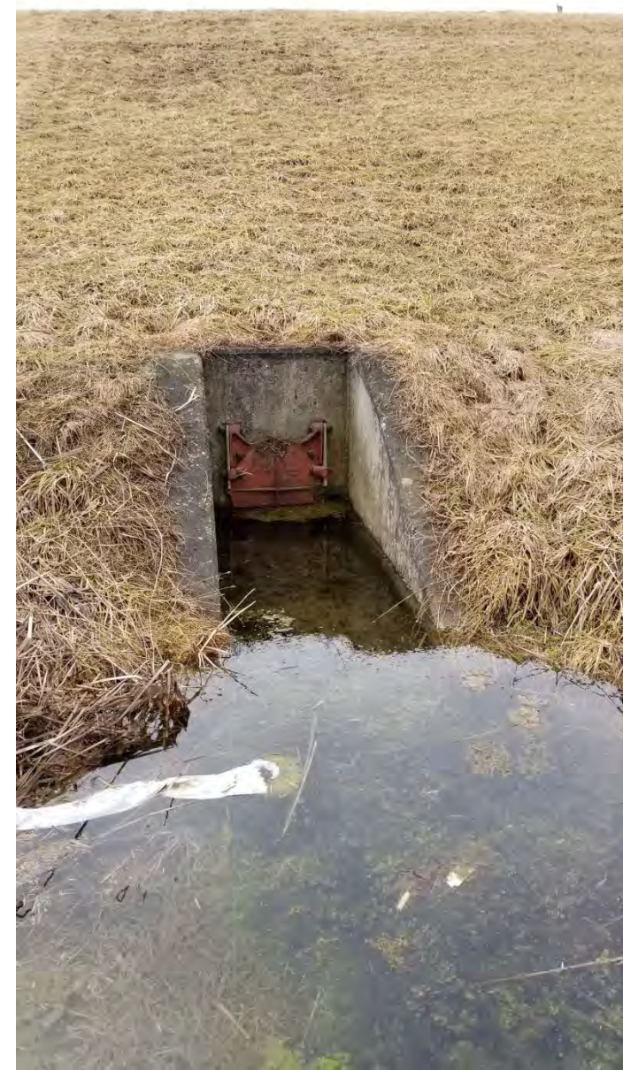
Typical outlet from stormwater system or toe drainage from land side of dyke
