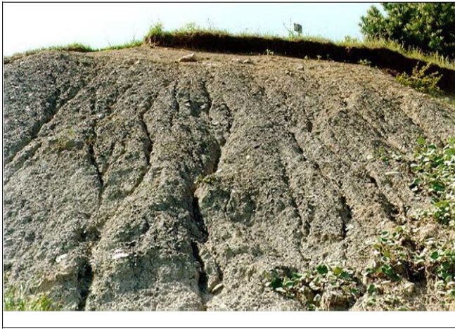
Figure 9 Rill erosion forms narrow channels on the face of a slope (left image) and can lead to more pronounced gully erosion over time (right image).
