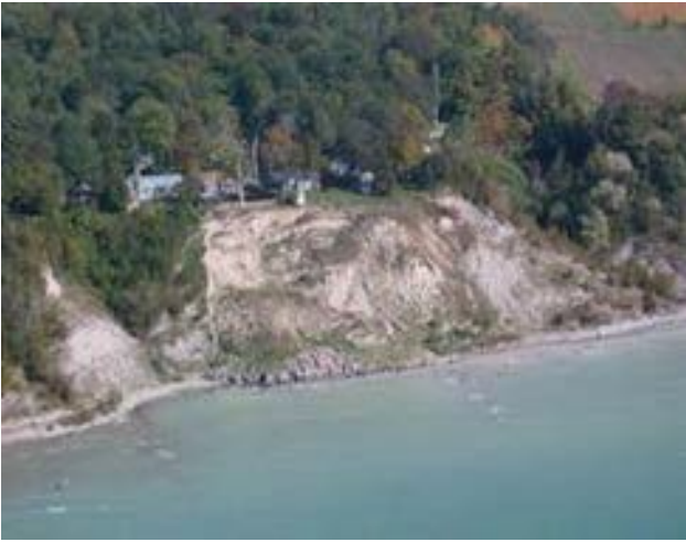
Figure 3 Bare slope areas exist where slopes are too steep for vegetation to take root and / or where a recent slope failure has occurred.
