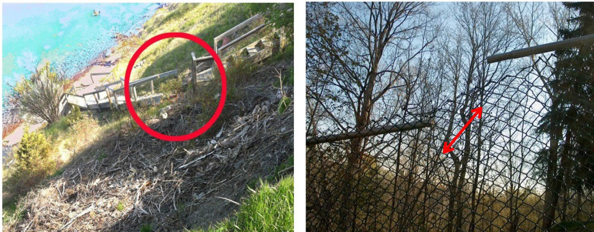
Figure 7 Other indicators of slope instability can include breaks in stairs and fencing.
