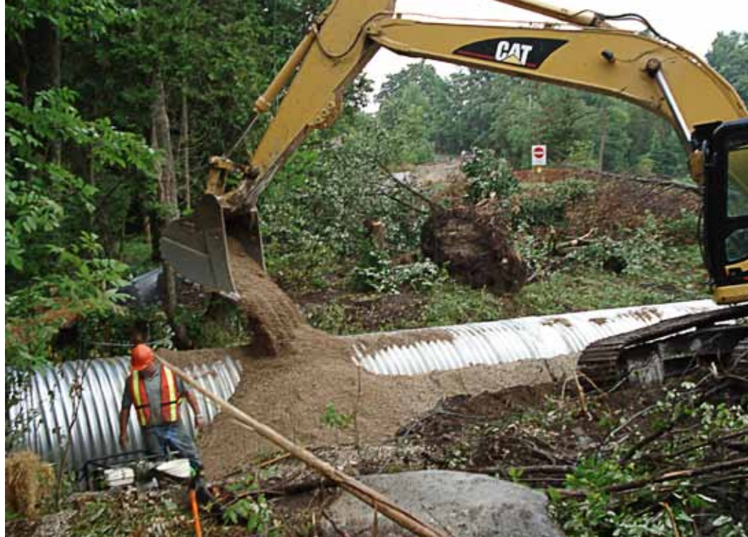
Culvert installation in Town of Chesley.
