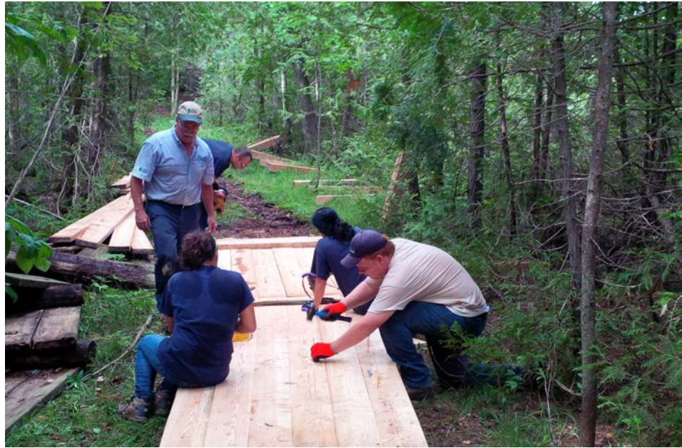
Staff work on the construction of a new boardwalk system at Schmidt Lake, part of the Greenock Swamp complex.
